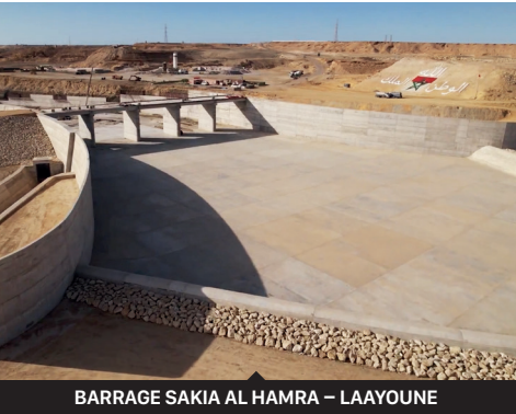
BARRAGE SAKIA AL HAMRA – LAAYOUNE
